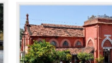
VICTORIA WATER WORKS In 1903, given by Maharaja of Pithapuram, who donated 40 acres of land for the municipality for drinking water.
