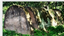
AIR RAID SHELTER Built in 1942 C.E during Second World War by the British government as a shelter for the soldiers to hide during bombing by air raids.
