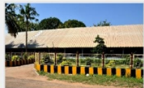
JNTU CIVIL BARRACKS Built in year 1946 and exhibited on July 16 th 1946 by Hon'ble T.S. Avinashilingam, education minister, government of Madras.
