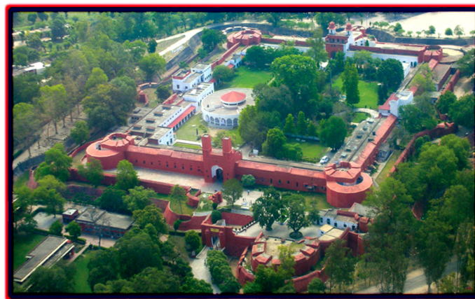
Figure 3: (An aerial view of Maharaja Ranjit Singh Fort Phillaur, presently housing Panjab Police Academy.)
