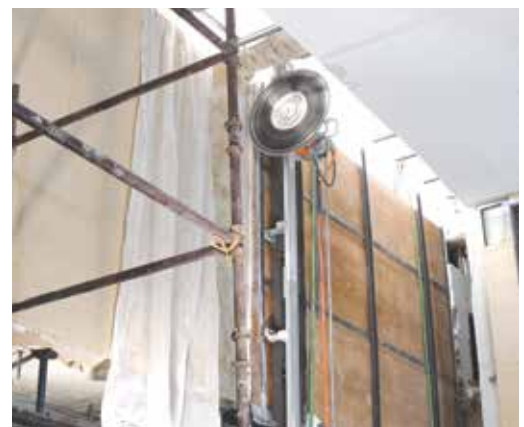
The saw used in diamond cutting; was used for the cutting the dummy and the original mural walls
