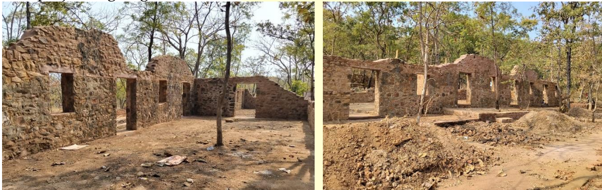
Ongoing Restoration of POW Camp, Delawadi – Bhopal Chapter
