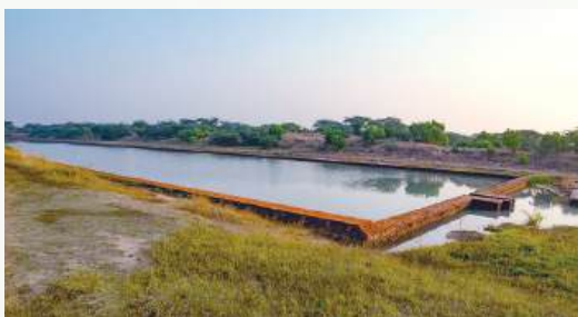
Dockyard at Lothal (Source: Open website)
