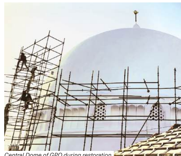
Central Dome of GPO during restoration
