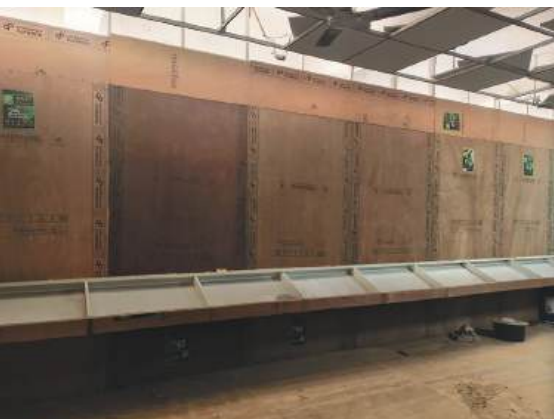
Wall paneling work is under progress at site
